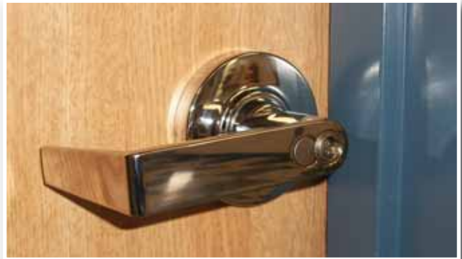
CyberLock padlock on office door lock.
